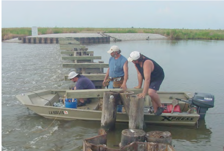
Workers repairing the Big Dam Weir Platform
